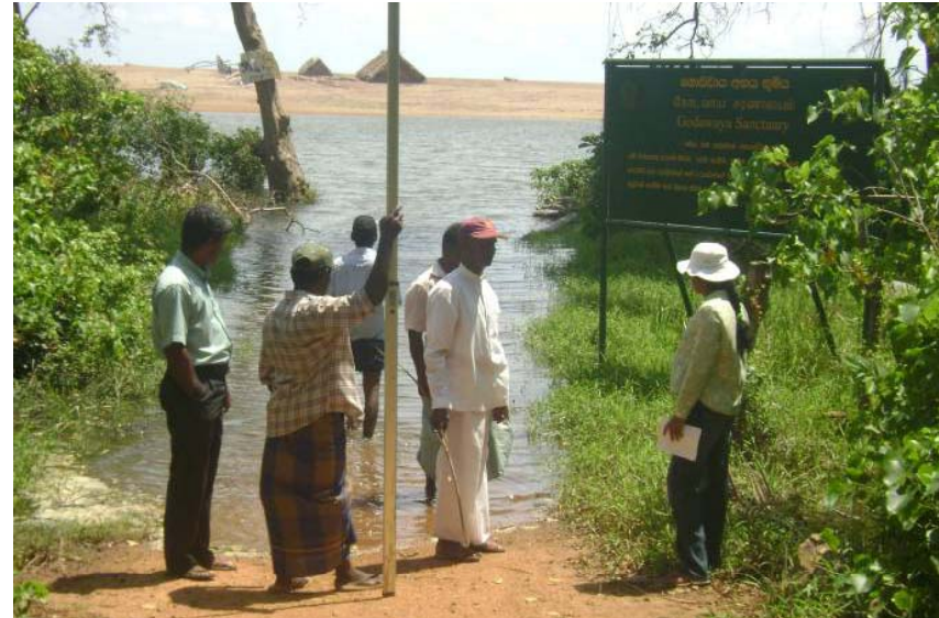
Installation of flood gauges
